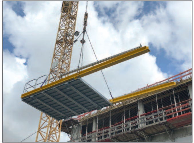
Transport to the site by crane
