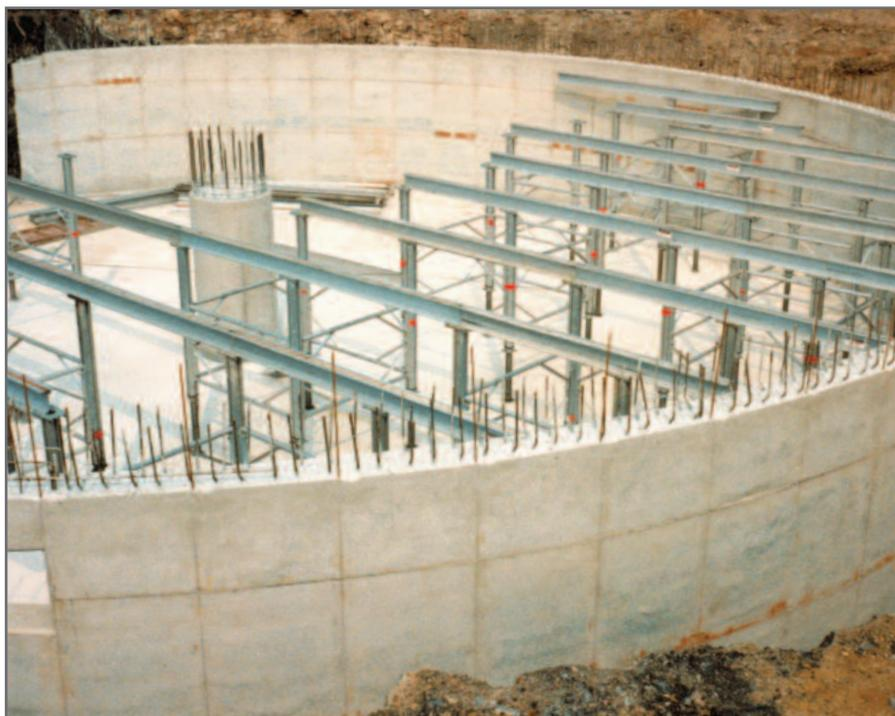
*110 heavy duty aluminium props – they replaced the planned 310 steel props*
