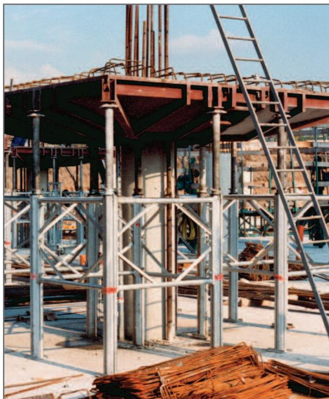
*H-frames for stabilizing special formwork of mushroom head*
