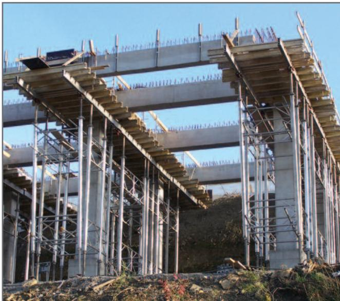
Shoring towers for insitu concrete main girders with supported secondary girders made of prefab elements.
