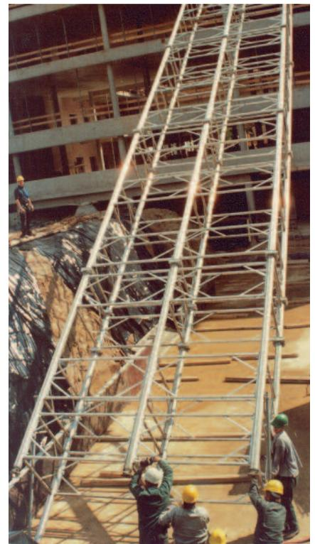
Tower unit consisting of 6 props, erected upright in one piece
