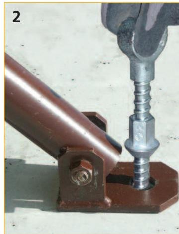
2. Screw bolt into the anchoring ground.
