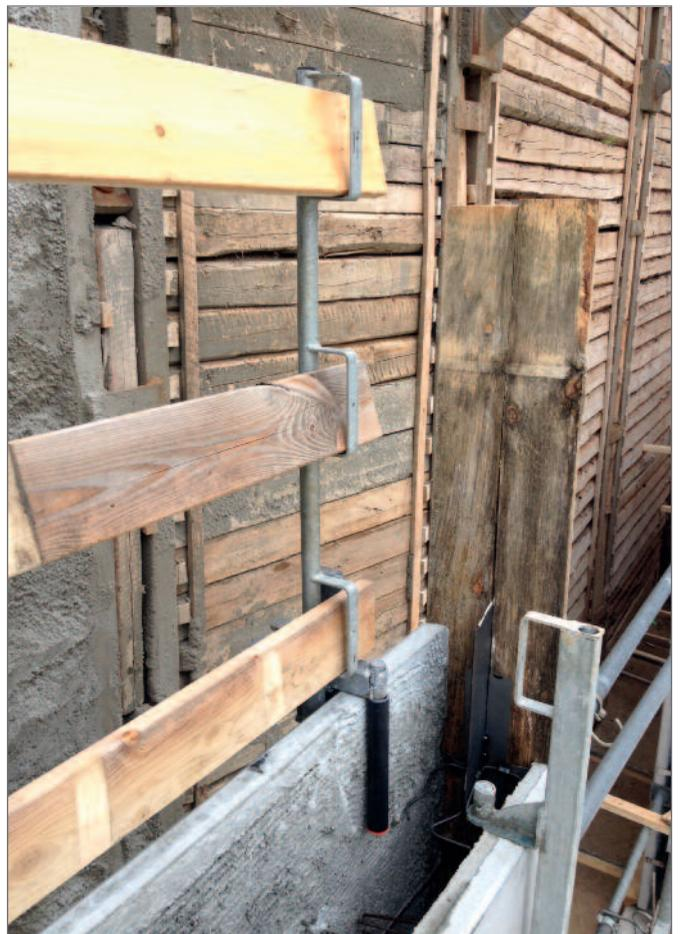
Use in combination with the twin wall concreting bracket / -working platform as protection towards the opposite side.
