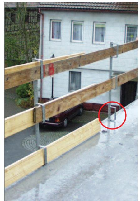
side railing post stuck into plastic tubes
