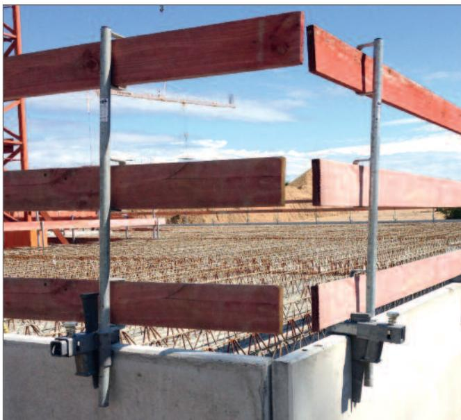
Use as a single part at the outer wall with already laid slab.
