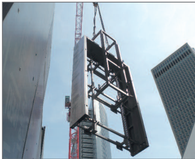
The formwork is transported to the place of use
