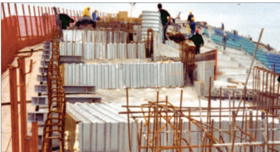
Special casings to produce cavities in the slab, especially adapted variations for different slab inclinations
