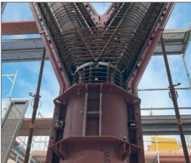
Special Y-shaped formwork combined with round column formwork
