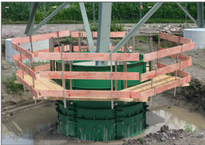
Special-purpose formwork for mast foundations before delivery
