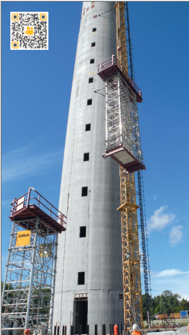
BV Thyssen Tower: Steel construction in combination with aluminium towers
