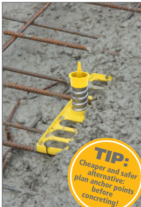
Before concreting: Installation-Kit with alignment D&W 20 mm
