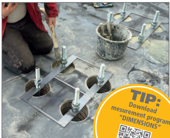
Grouting the anchor rods with anchor grout. Shown here: installation of a quadruple set using an installation template.
