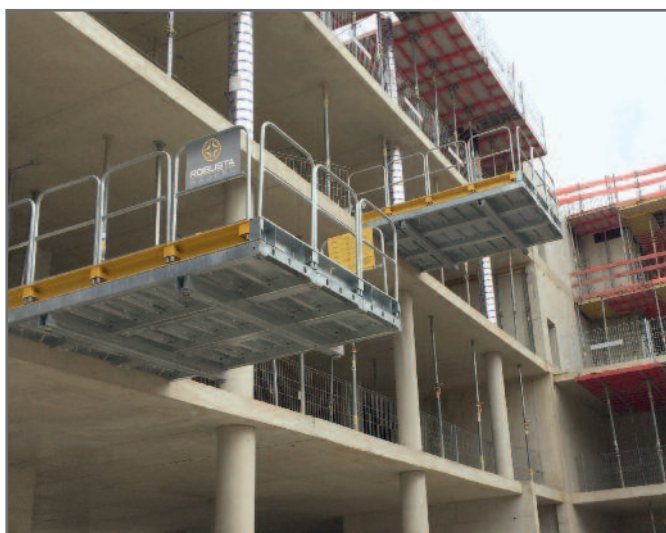
Mounting by way of anchoring in the slab
