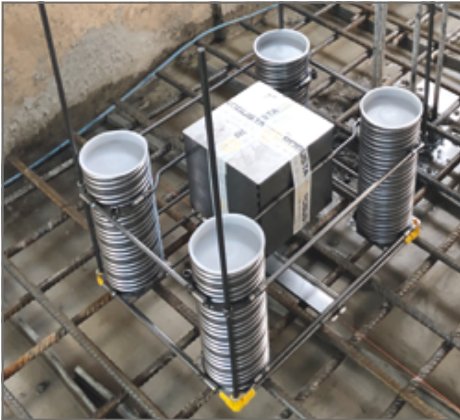
Fixing the mounting frame to the bottom reinforcement layer with wire. Complete Quad-Set with shear key and alignment plate.
