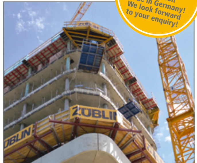
BV SKY Bietigheim: Special formwork platforms for precast elements
