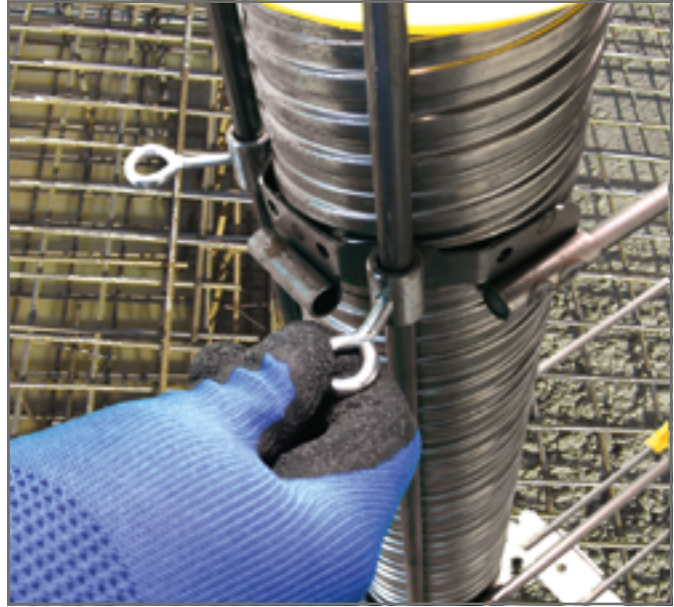
Fixing of the anchoring sets on the vertical rods of the mounting frame after setting the correct height. This can be done before or after the top layer of reinforcement is laid.
