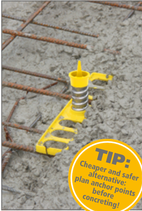
Before concreting: Installation-Kit with alignment D&W 20 mm
