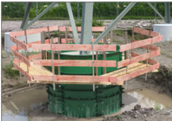
Special-purpose formwork for mast foundations before delivery
