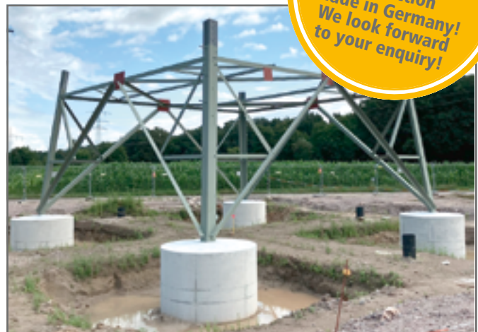
Result after stripping work
